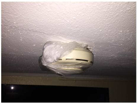
A covered (and by extension, disabled) smoke detector represents a fire risk to occupants of the room and to the rest of the motel and its occupants.
