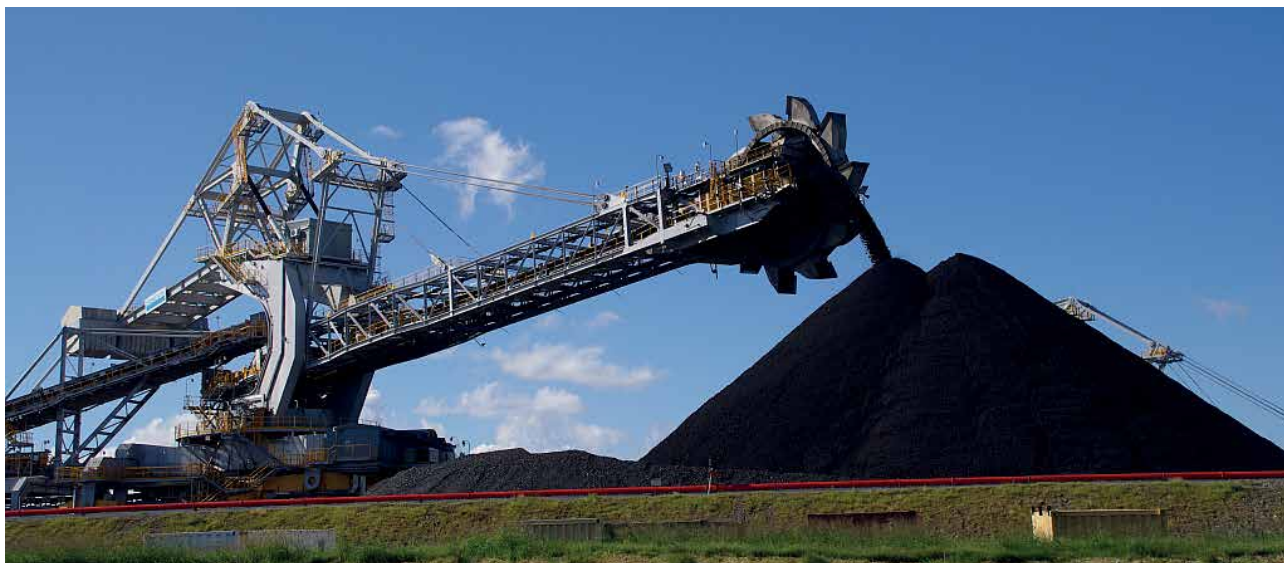
Figure 6: Coal loading at Korragang Island, NSW.
