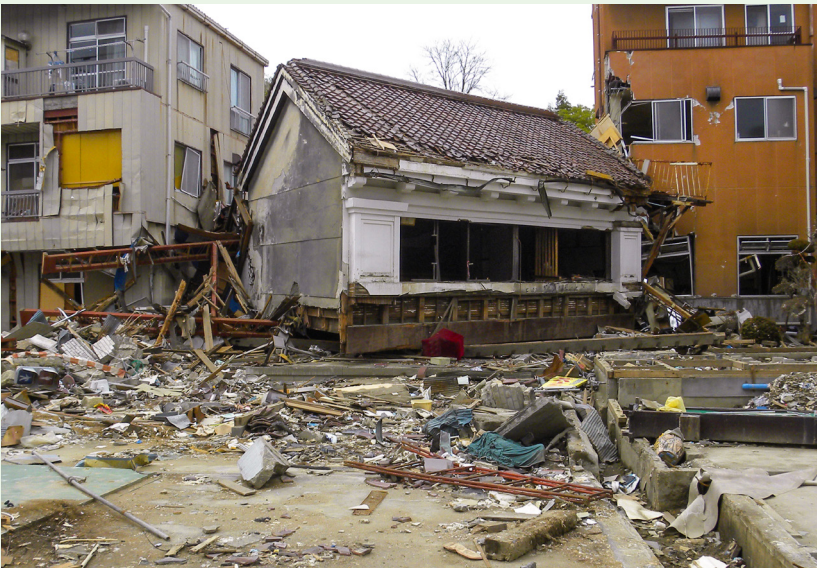
Building collapse caused by tsunami in eastern Japan, 2011. Photo: Board of Miyagi prefecture.
