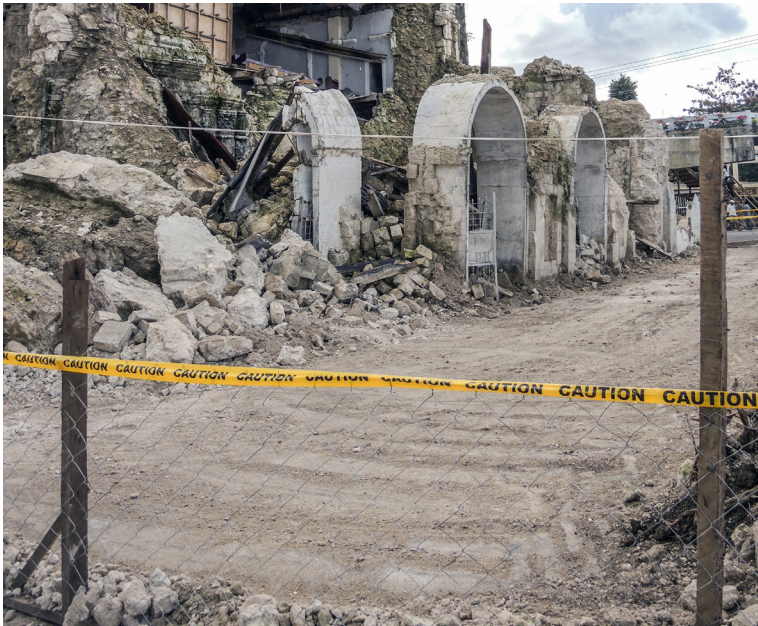
Barriers and caution tape help to warn people and secure a heavily damaged church in Philippines, 2013. Photo: Aparna Tandon, ICCROM.
