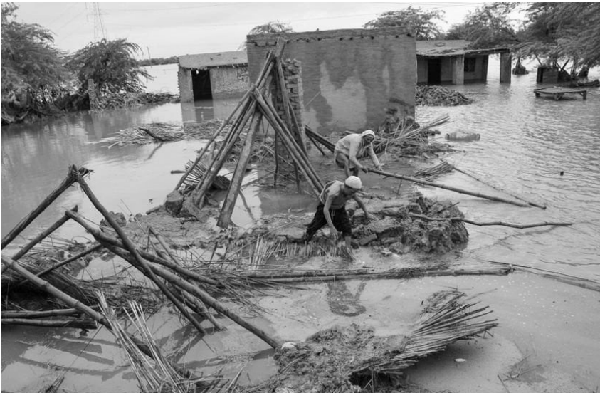
A large number of public and private properties and infrastructure were damaged during the mid-year flash floods.
