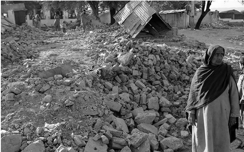
Officials of the Capital Development Authority (CDA) reportedly destroyed over 100 makeshift homes in a slum colony housing Christians in Sector H-9 of the capital.
