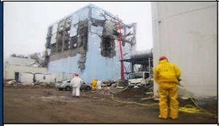
Figure 12: Fukushima's Unit 4 after a hydrogen explosion rips apart the 3rd, 4th, and 5th floor. Photo courtesy of Forbes: http://www.forbes.com/sites/williampentland/2013/12/30/yakuza-gangsters-recruit-homeless-men-for-fukushima-nuclear-clean-up/
