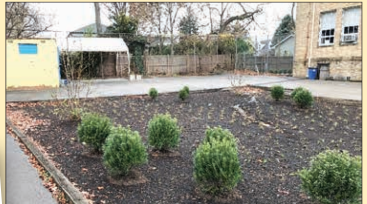
Above: The installation of a 1,750 square foot rain garden at the location of an old playground.
