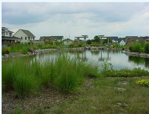
*A stormwater collection pond in a Minnesota neighborhood captures and temporarily stores stormwater runoff.*
