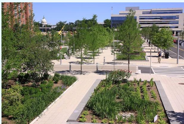
*Canal Park in Washington, D.C., incorporates cisterns, rain gardens, and bioretention tree pits to capture, treat, and reuse stormwater.*
